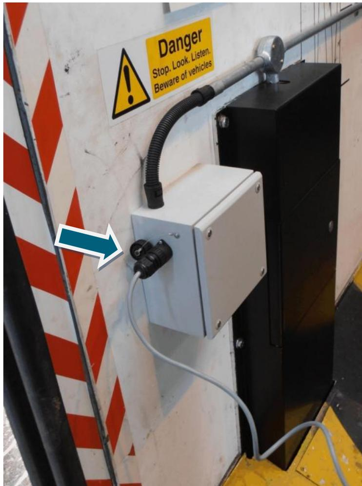
2:7 Electric Winder Remote Control Connection
